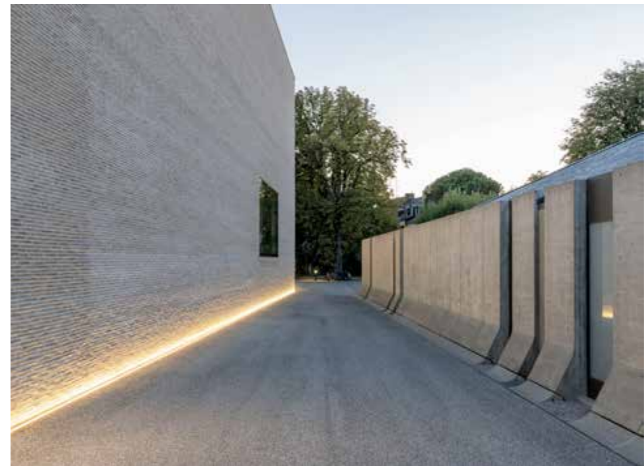
Different shades of gray: a dynamically staged passageway between the existing structure and the new building
